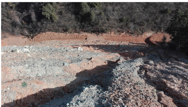
Fig. 1 Photograph of a typical engineering spoil heap in a clay loam area
